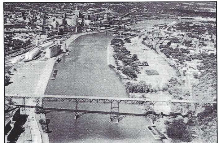
1962 -- Excavation if process at upper end of Harriet Island, part of the seawall and redevelopment program and possible future site for the new St. Paul Yacht Club marina.
