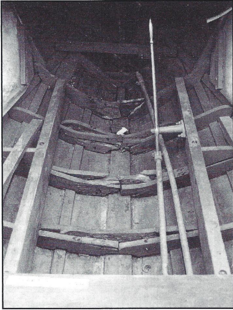
Serious damage to the bottom frames is evident from an unknown incident.
