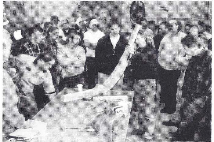
Mark Sauer Shows the assembly of keel to stem to gripe.
