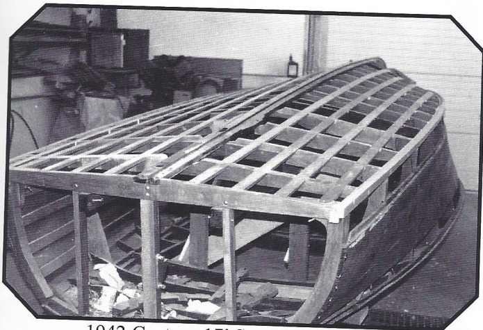
1942 Century 17' Sea Maid showing restored frames and battens
